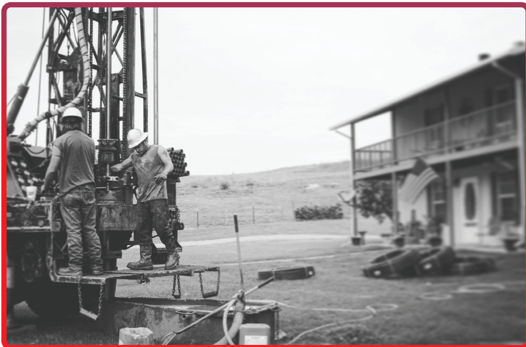
A loop installation financed by CKenergy's Geothermal Program
